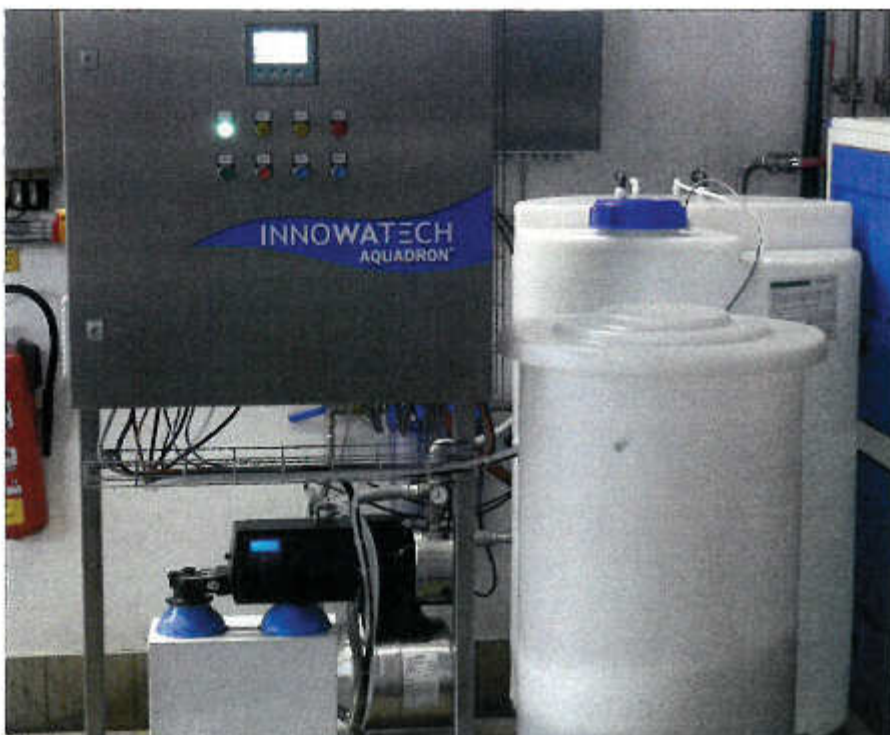
Innowatech Aquadron SGX allows for the generation of anolyte right at the application site.
